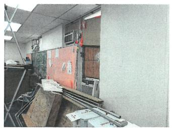
classroom side of the classroom walls. More efficient and securly mounted HVAC units may be required in these classroom. If these units remain, the exterior or outside wall mounts will need to be reinforced.
